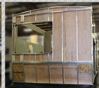
Double welded aluminum cage construction in walls and floors.
